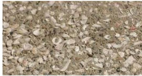
FOUNDATION CEMENT TABBY STUCCO
