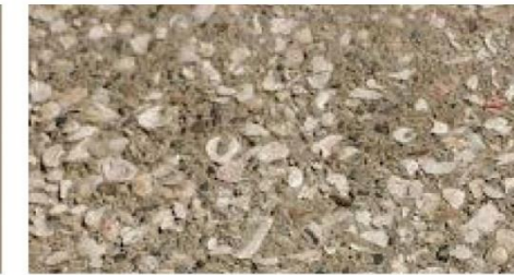
FOUNDATION CEMENT TABBY STUCCO
