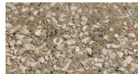
FOUNDATION CEMENT TABBY STUCCO
